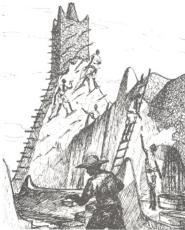
Masons were very important workers in West African towns and cities. Masons here build the masjid at Sankore. They use ladders to reach the top of walls. Towers, or minarets have wooden beams built into them, making them look like porcupines. That way, workers can reach every part of the walls. That is important, since the building needs a new coat of mud plaster each year after the rainy season.
